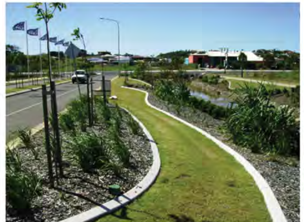
'Smarter' rather than wider, this set-back at Mackay combines landscaping elements to slow and trap the movement of runoff towards the waterway.
