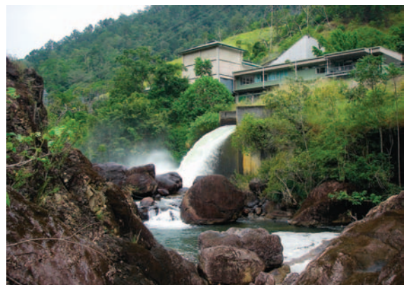
An impressive scene – the Tully River Tail Race flows when water from the turbines is discharged into an open concrete sluiceway
