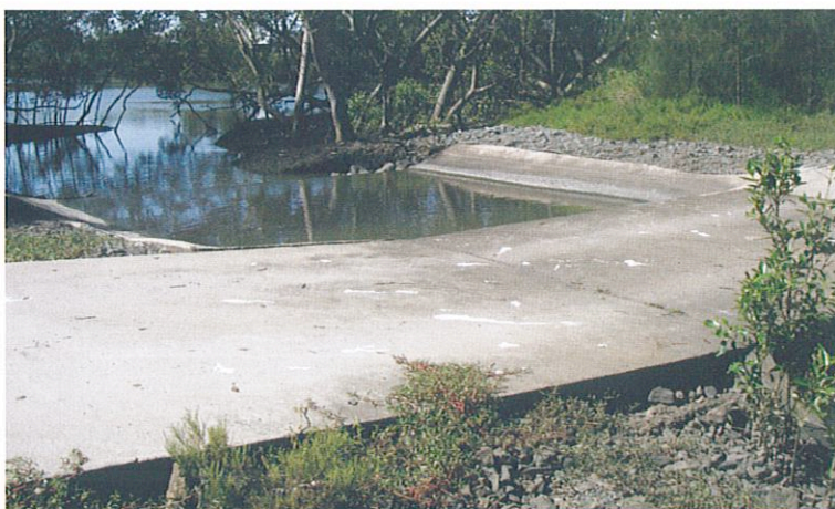
Crossings and culverts can significantly impact flows in mangrove lined creeks
